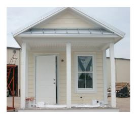
The Park Model and Mississippi Cottage were designed to address the shortcomings of the travel trailer and mobile homes used by FEMA following large-scale disasters. Design priorities included energy efficiency, minimal environmental impact, safety, durability, and the ability to provide immediate (short term) yet permanent (intermediate and long term) affordable housing.
